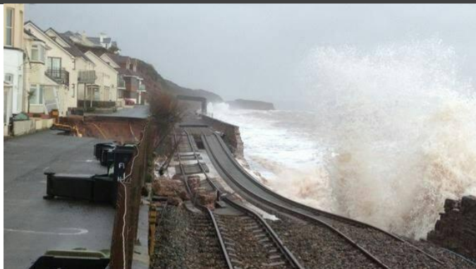
Storm surge UK Feb 2014 (Met. Office) Collapse of railway embankment in Dawlish
